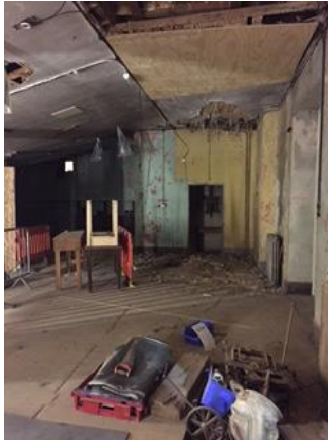
Image of under the theatre balcony
